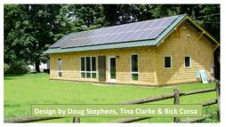
Attractive, small, sensible, **astounding** performance 1152 Square feet R40 walls, R100 roof, triple glazing, R30 slab (no basement!)
