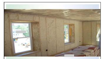
12" double stud walls 2x4s, 16" OC outer, 24" OC inner 0.5 lb/cf spray foam, R-4/in
