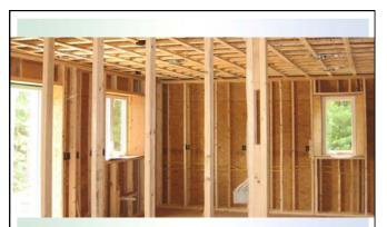
12" double stud walls 2x4s, 16" OC outer, 24" OC inner 0.5 lb/cf spray foam, R-4/in about R-45 total
